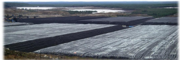
The Talvivaara Mine primary bioleaching heaps in the front and process water reservoirs behind.
